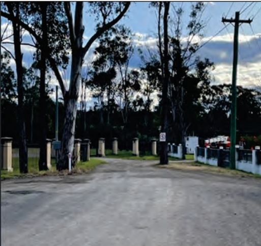
Photoplate 18: View of Site from Residents in the East, 2022.
