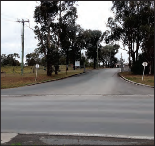
Photoplate 4: View of Site Entrance & Quarry from Greendale Road, 2024.
